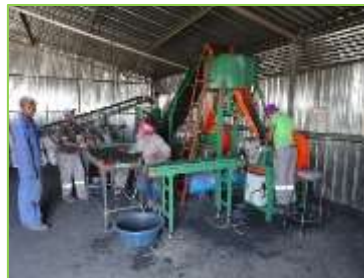
Picture 50: Small scale briquette production plant
