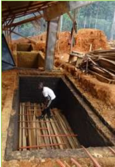
Picture 23: Mindourou Kiln – Filling operation
